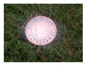
The term "monument," when used in reference to boundaries, indicates a permanent object which may be either natural or artificial. These brass objects are mounted atop a 40" high concrete pillar. The pillar is set into the ground, with only the monument and a small amount of the pillar protruding.
